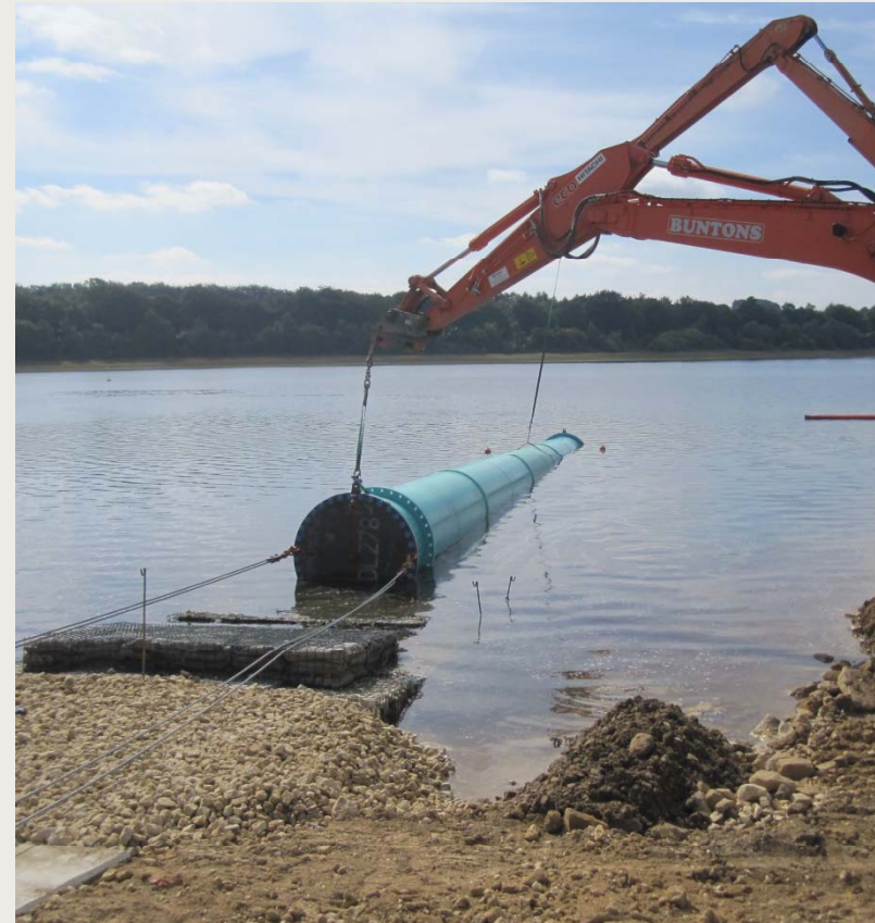
View of upstream siphon pipe being located onto pipe supports.
