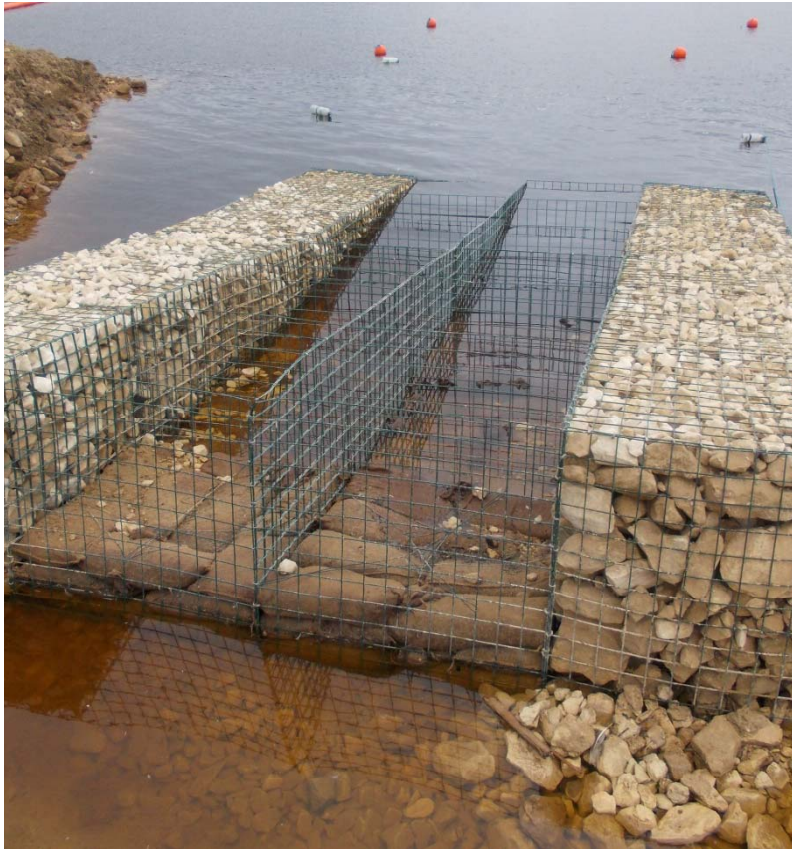
View of upstream supports during construction.
